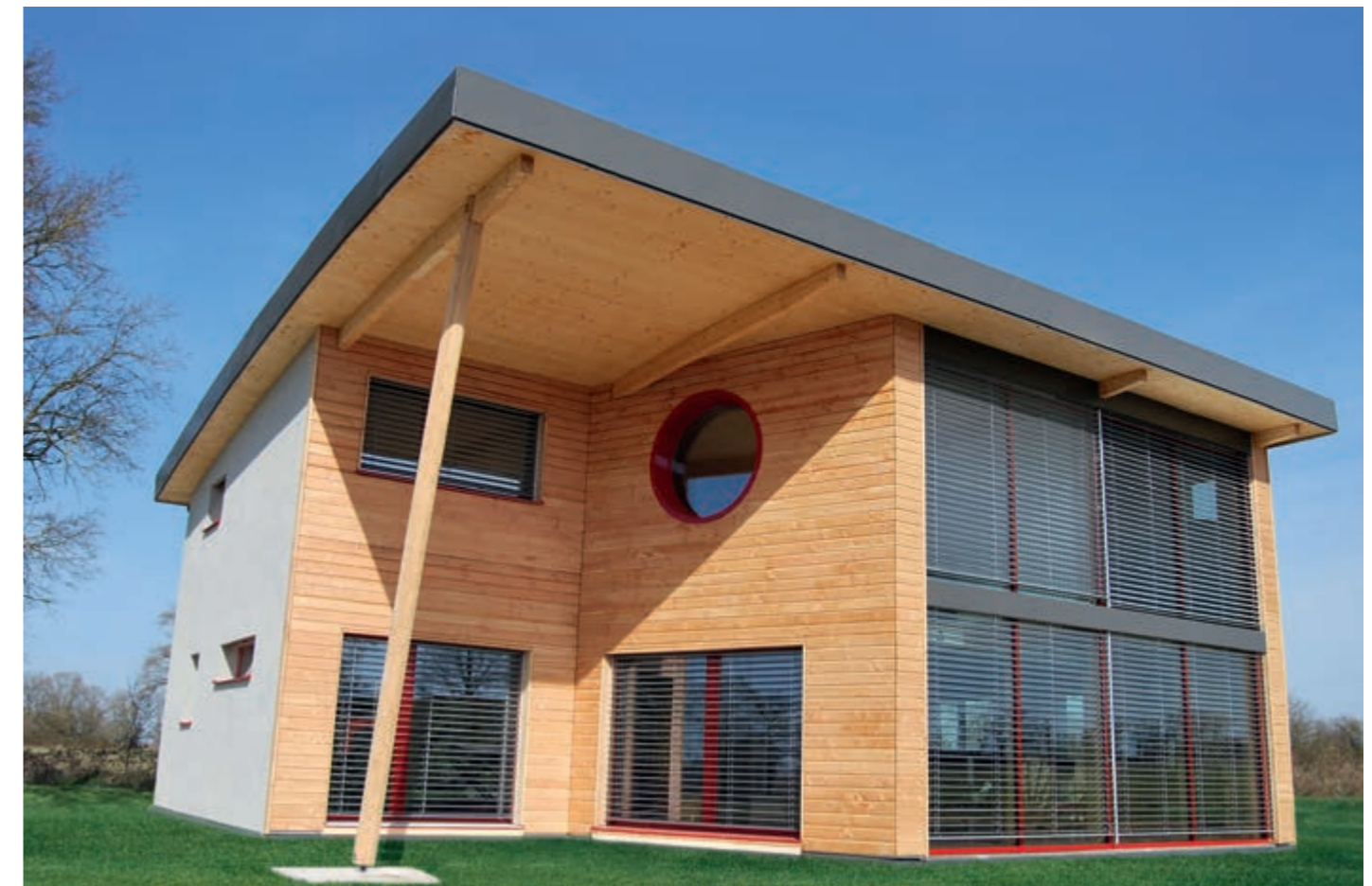
Single-family home in Bellac | Passive house, | Area: 117 m² | Thickness: 240 mm
